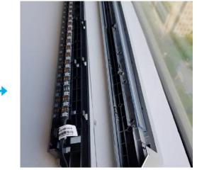
11. Once the strip is properly attached, pass the LED wire head through the square hole.
